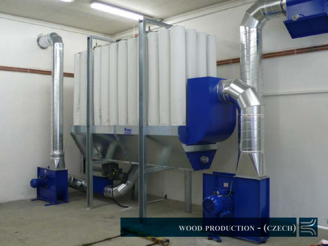
Machines designed for **large amounts** of non-explosive non-sticky **dust, small** waste and fumes. They are used as central dust extraction of grinding tables, blasting booths, milling and grinding machines, CNC milling machines, etc. Suitable for exhaustion of plasma and laser milling machines.
