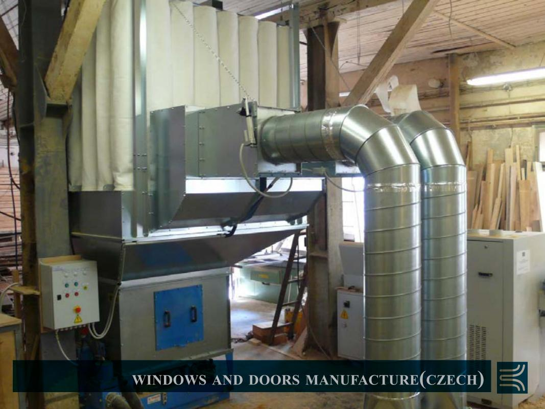
Cyklone is designed to capture larger particles of waste during extraction. The separator proves to be a **pre-separation** before the main filtration, **it catches up to 97% of waste**, which is able to ensure the **extension of the filter life**.
